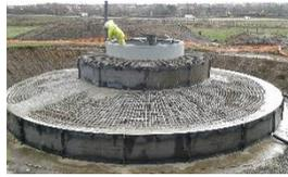
Once all shuttering was complete the turbine and substation foundations were poured on the same day, and stripped within 48 hours.
